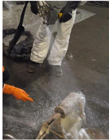
Figure 2: SGFRP strengthening process
