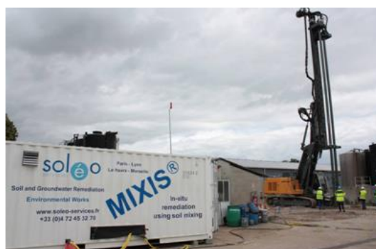
Figure 1: Figure illustrating the field remediation of a site contaminated by chlorinated solvents, by injecting zerovalent iron nanoparticles into the soil and groundwater by soil mixing (© Soléo Services company).
